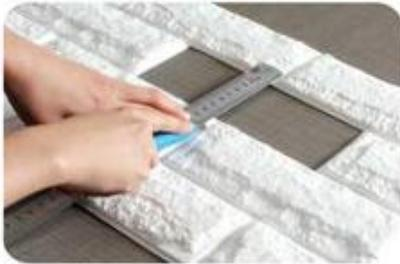
**1. Cut off the area that will be applied a brick of different color before adhering the panel.**
