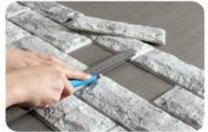
**3. Cut the brick sheet of the other color to match the Foam brick sheet cut before.**
