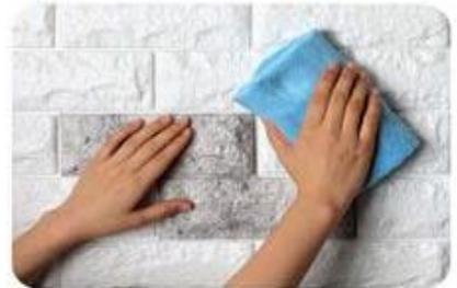
**6. Smooth out the surface neatly after application and clean off the surface with dry cloth.**
